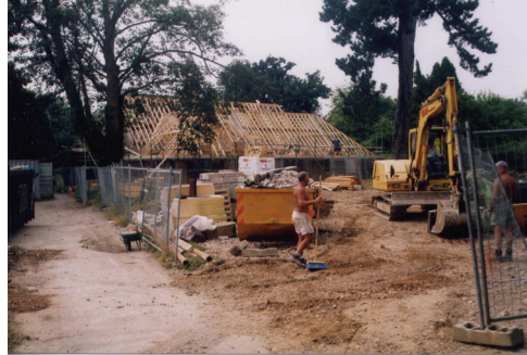
9 August Roof beams in place
