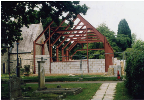
1 June The walls begin to appear
