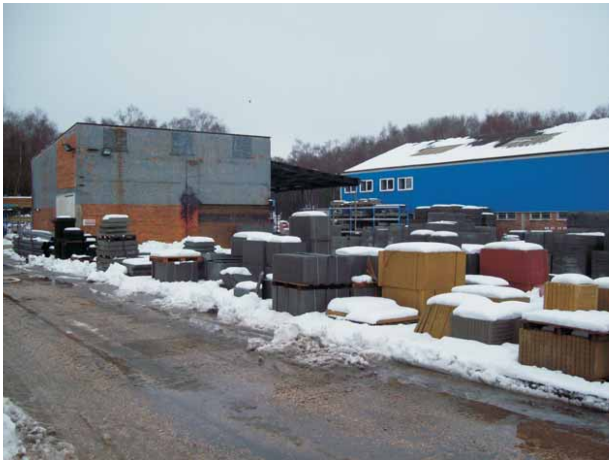
Plate 5: Main and ancillary building from the south east
