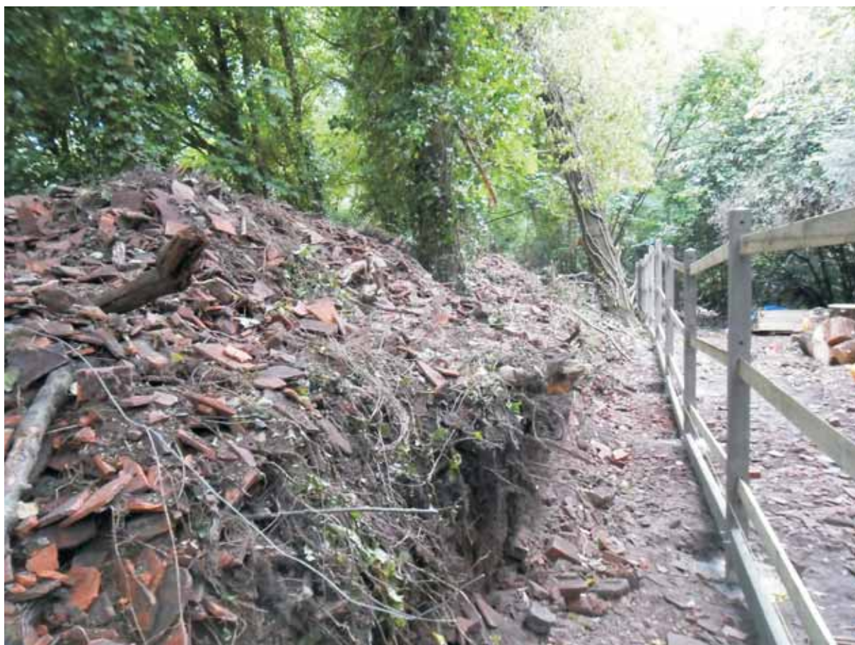
Plate 10: Creation of a new fence line through the bank at the northern boundary of the site (June 2011)
