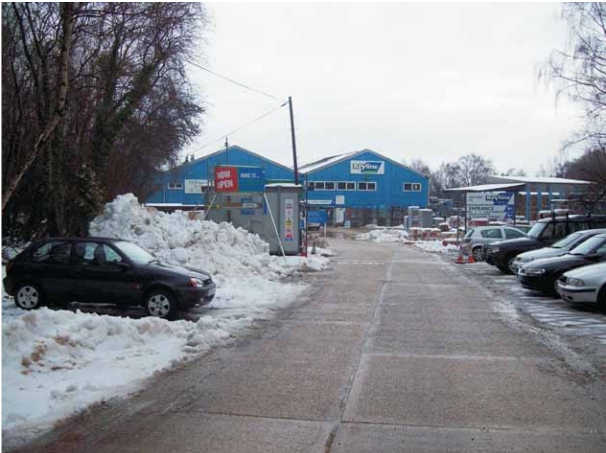
Plate 4: Main building from the west
