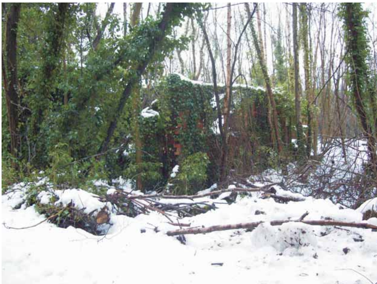
Plate 6: Small structure on the higher ground north of the yard area
